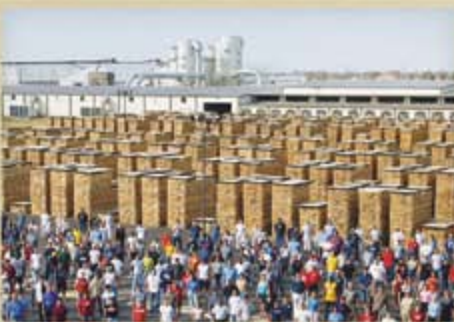
View of manufacturing plant from lumber stack yard.
